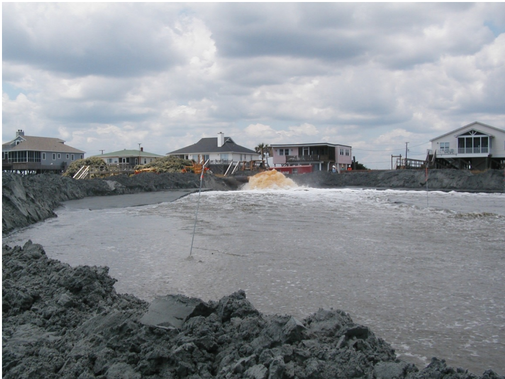
Figure 4-1. Example of beach fill construction (Folly Beach, SC).
